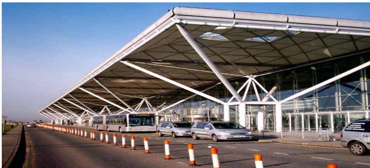
Fig.-2 Stansted Airport displays the use of steel modules to provide long span and other design features that enhance its sustainability.
