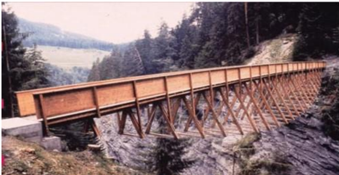
Fig.-1 Traversing Bridge showing the use of locally available timber to enhance its sustainability.
